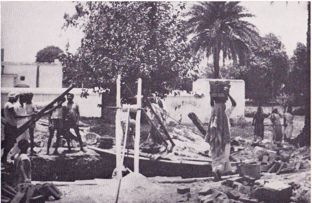
Bricklaying in new irrigation well at Yogoda Satsanga headquarters, Ranchi. Ropes and pulleys haul up baskets of dirt or buckets of water to keep hole clean and dry. White wall ( in background ) encloses garden patio.
